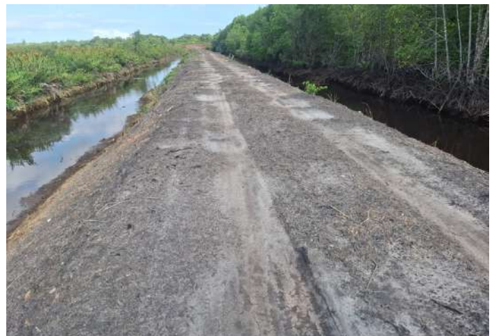
A bund constructed at Ladang Mamahat (Terusan Division).
